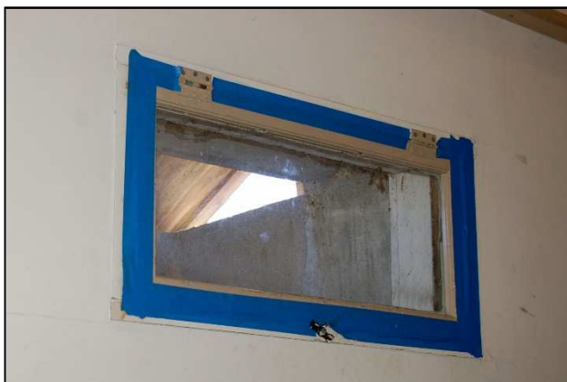
Figure II-11: Replacement lower level sash
