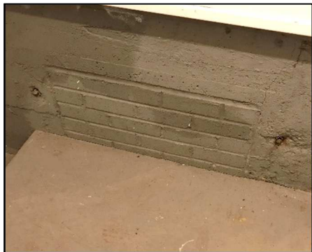
Figure III-24: Infilled window
