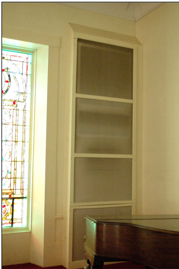
Figure III-60: Mechanical ductwork enclosure
