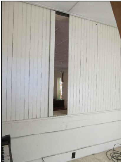
Figure III-71: Beadboard sliding panels, opening to Sanctuary
