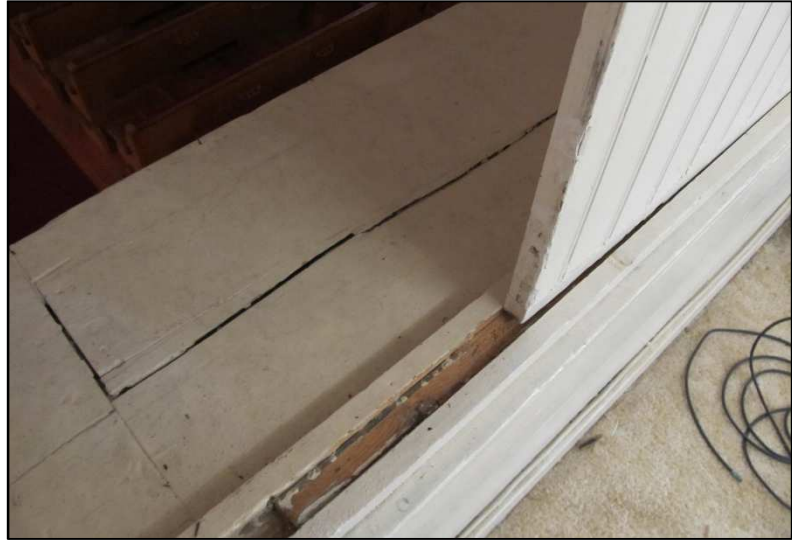
Figure III-70: Wooden track for beadboard sliding panels
