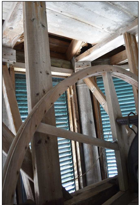
Figure III-87: Rotted beams at Lantern
