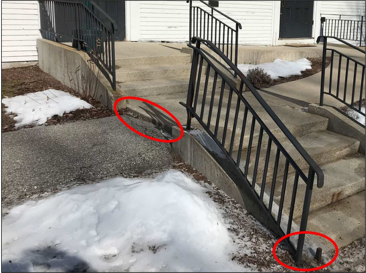
Figure III-3: Disconnected railing and lip at intersection between asphalt and concrete at ramp
