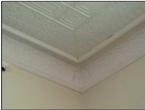
Figure III-54: Steel crown molding
