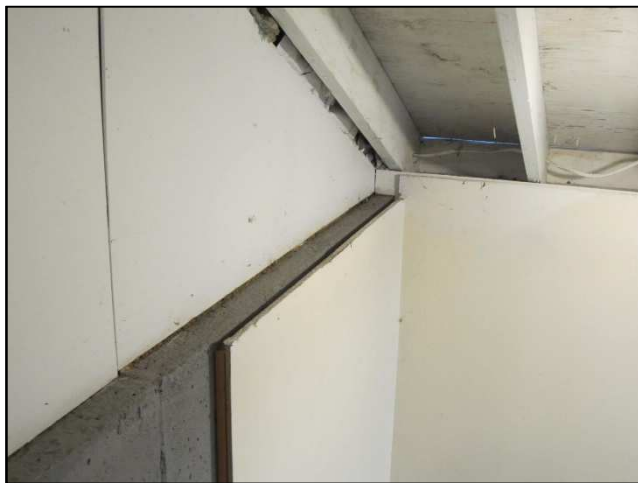
Figure III-25: Exposed roof structure at egress enclosure
