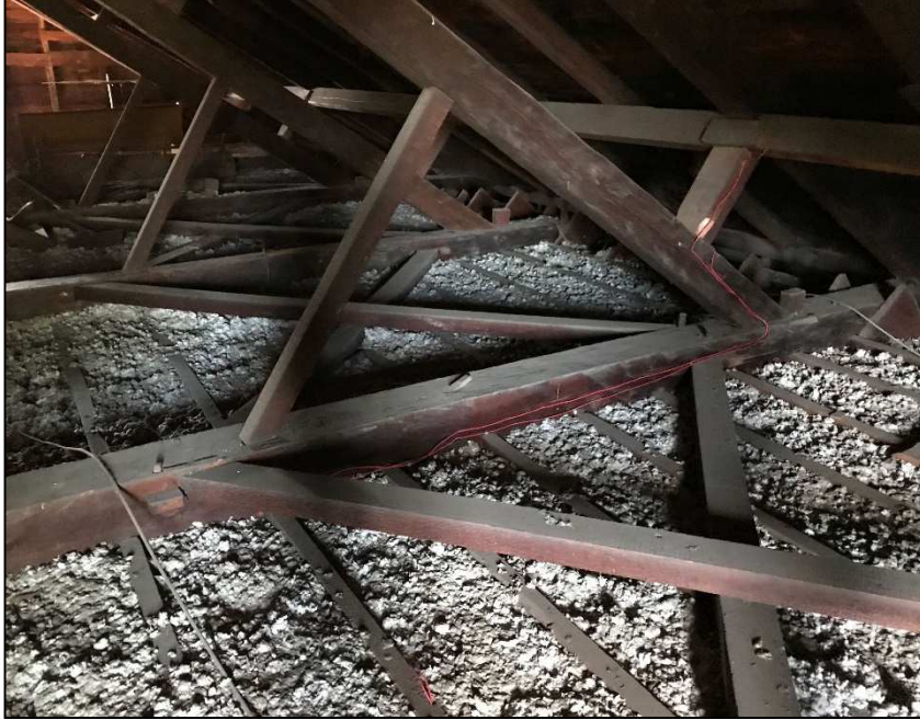
Figure II-49: X-braces in floor of Meetinghouse attic
