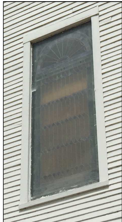
Figure III-6: Upper level stained glass window with plexiglass covering
