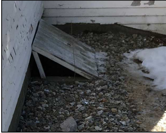
Figure III-11: Typical window well & cover
