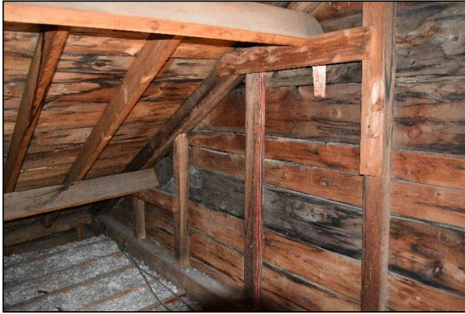
Figure II-51: Framing system of 1867 vestibule addition
