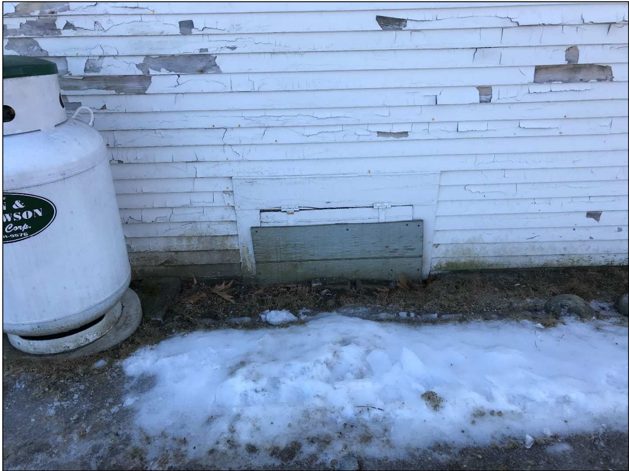
Figure III-4: Grade at the north elevation of the Meetinghouse has risen above the bottom clapboards
