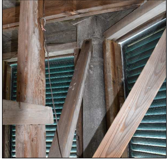
Figure II-61: Modern bracing
