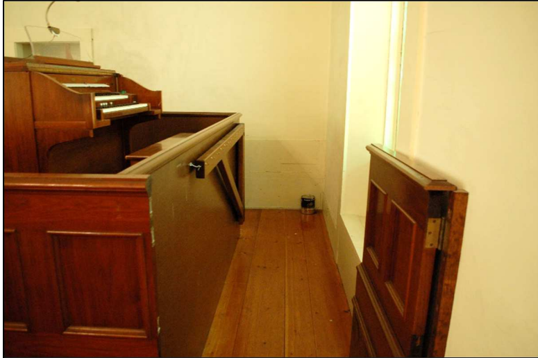
Figure III-59: Mahogany wall panels with integrated egress path
