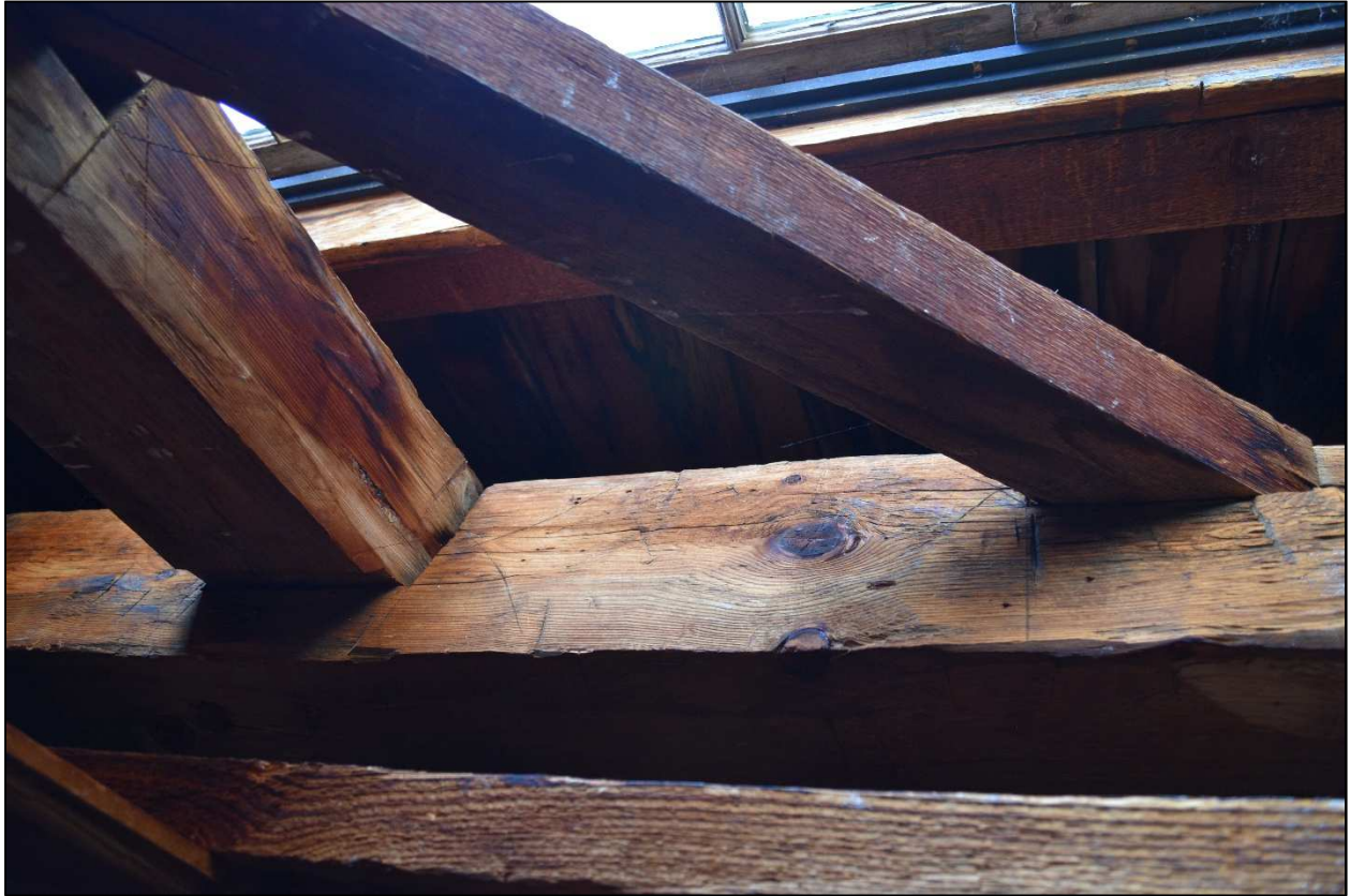
Figure II-56: Square rule framing marks outside of clock room
