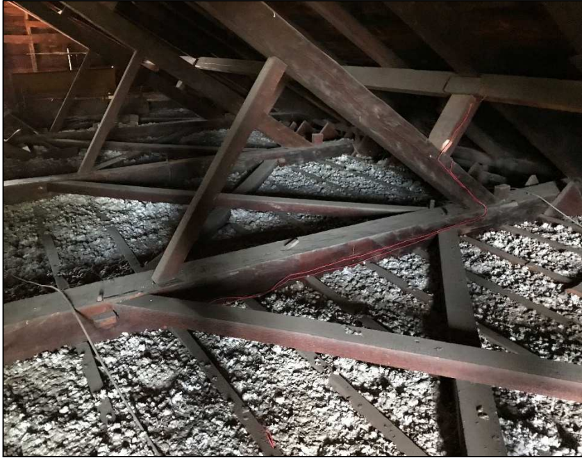
Figure II-49: X-braces in floor of Meetinghouse attic
