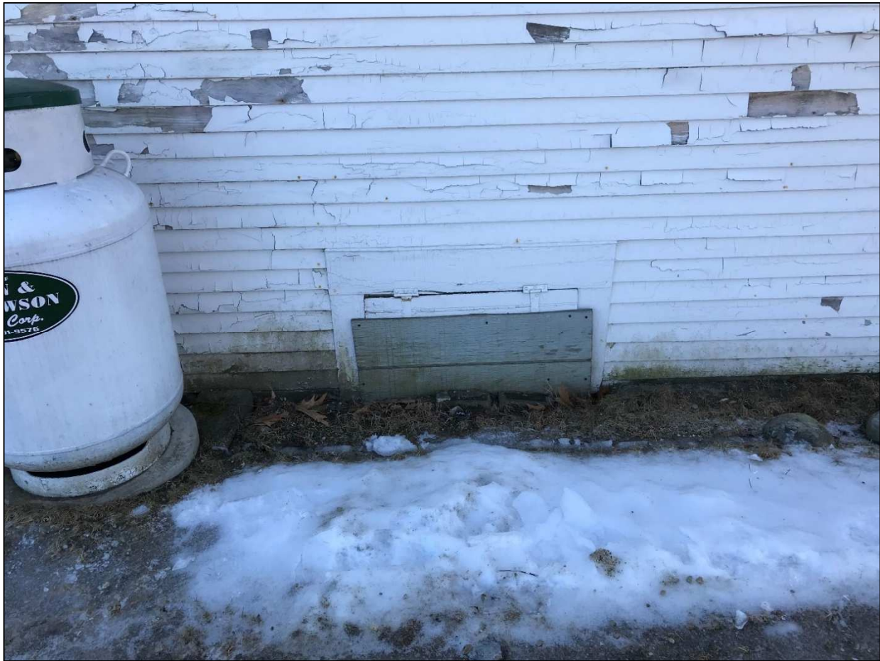
Figure III-5: Grade at the north elevation of the Meetinghouse has risen above the bottom clapboards
