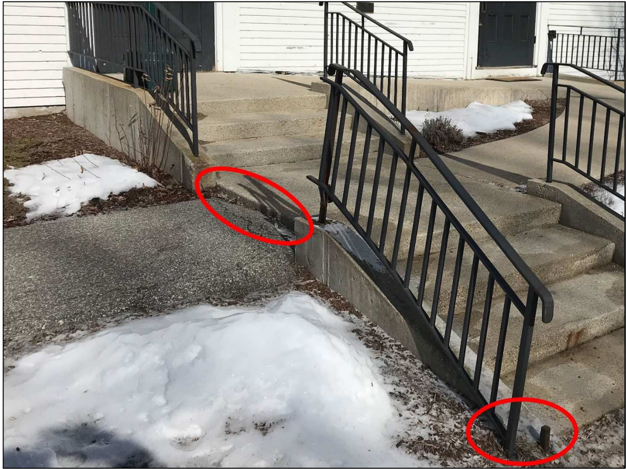
Figure III-6: Disconnected railing and lip at intersection between asphalt and concrete at ramp
