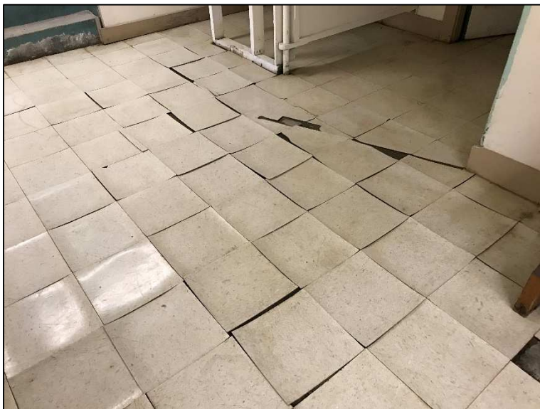
Figure III-18: Tile floor of the Community Room with moisture damage
