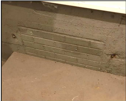
Figure III-26: Infilled window
