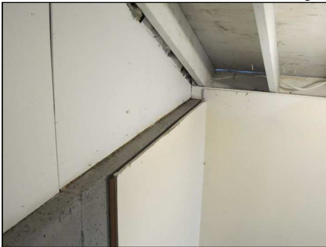
Figure III-27: Exposed roof structure at egress enclosure
