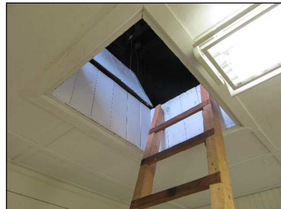
Figure III-76: Access hatch to Attic
