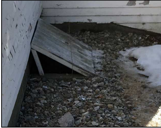
Figure III-13: Typical window well & cover
