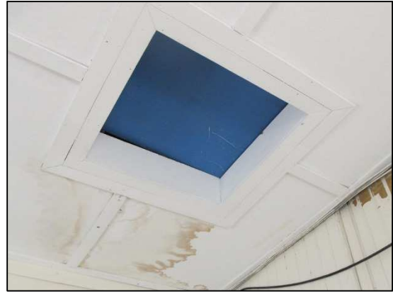
Figure III-74: Unused access hatch to Attic
