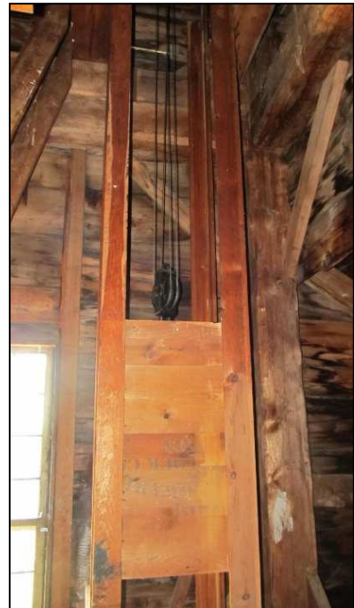
Figure III-81: West counterweight
