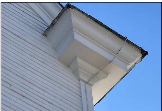
Figure III-15: Roof fascia & soffit detail
