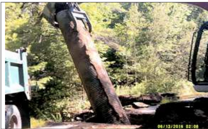
Old Steel Culvert
