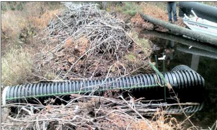
These new culverts don't hurt the beavers in any way but are supposed to let the water through preventing flooding from beavers plugging culverts under the roads. With any luck, they will solve some of our beaver problems. We spend quite a number of hours clearing culverts due to beaver so we are hoping that these culverts work the way they are supposed to.
