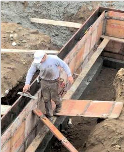
*Bill Harper, owner of West Rindge Building, takes a moment to measure the foundation wall prior to pouring the cement.*
