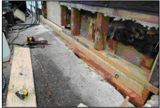
New sill installed
