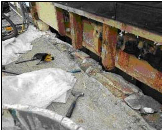
20 ft of the sill was removed
