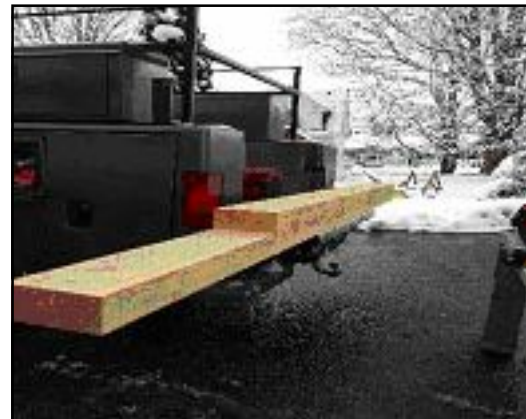
New sill with half lap joint
